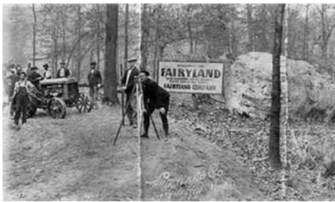
Figure 14. Surveying the Fairyland Club - https://lookoutmountain.club/HistoryOfFairylandClub
