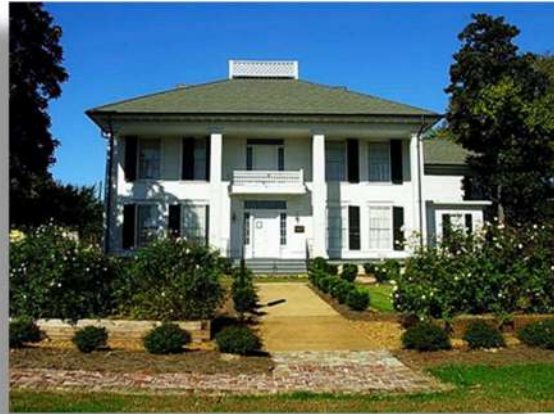
Figure 80. Historic Marsh House
