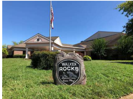
Figure 42. Walker Civic Center Campus at U.S. 27, Rock Spring, Ga.
