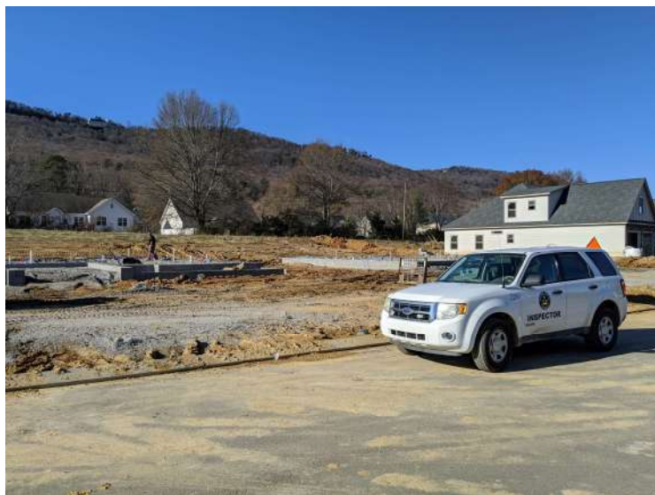
Figure 24. New Home Construction in Walker County
