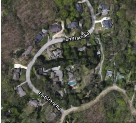
Figure 56. Fort Trace Road, at the City of Lookout Mountain
